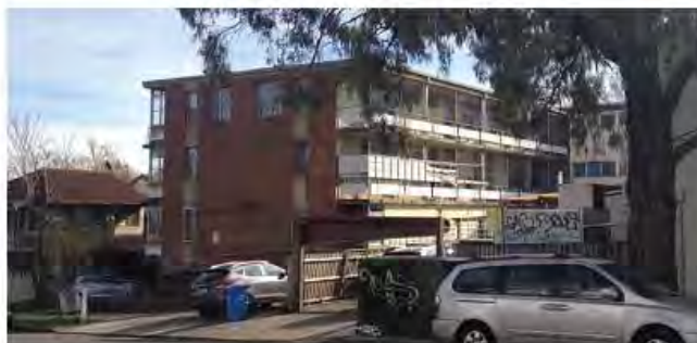
Figure 2.05: Site 2 – Carlisle Street location
