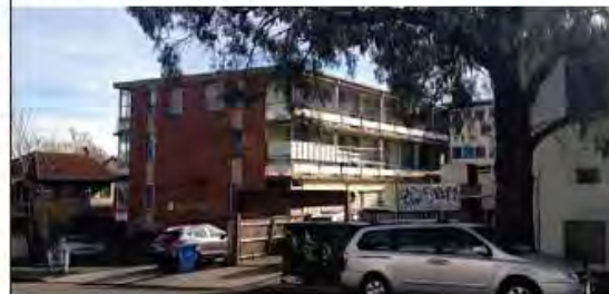
Carlisle Street – building in poor condition, unsafe
