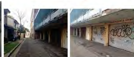
Rear lane, owned by LinkingCare – poor amenity, security + safety issues. It provides access to tenements
