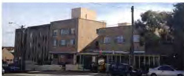
Figure 1.01: Site 1 - 17 Marion Street - Antaresby House
