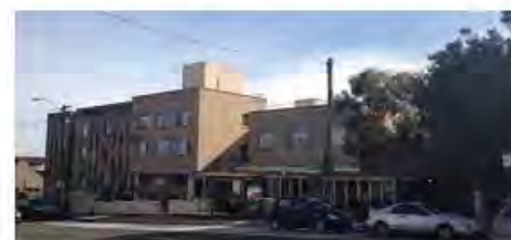
Marion Street - existing built form
